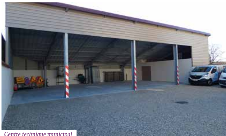
Centre technique municipal
